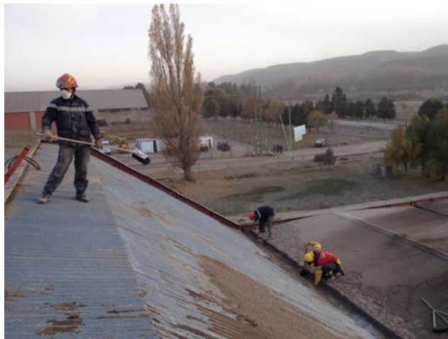
Volunteer firefighters work to clean ash from roofs in the town of Junín de los Andes, Argentina, following the April 2015 eruption of Calbuco volcano in Chile. Note the PPE worn by workers, the dry methods of clean-up, and workers staying well apart. Photo credit: Volunteer Fire Department, Junín de los Andes.
