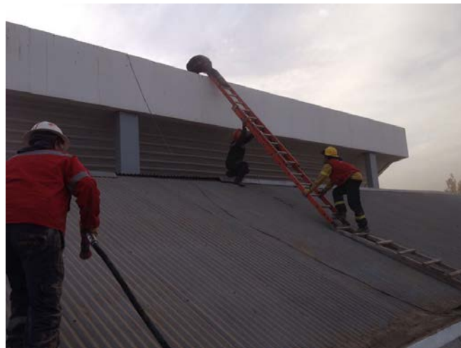
Use of ladders on roof for more secure footing during ash clean-up operations, Junín de los Andes, Argentina. Photo credit: Volunteer Fire Department, Junín de los Andes.
